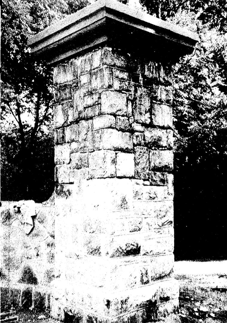
**CONCRETE CAP IN PLACE:** This is one of the new concrete pillar caps formed from a hand-shaped plywood mold. Its curves, grooves and lines are perfect. The stonework at the bottom of the pillar has been newly cemented. That at the top remains to be completed after the old mortar was chipped out by hand.
